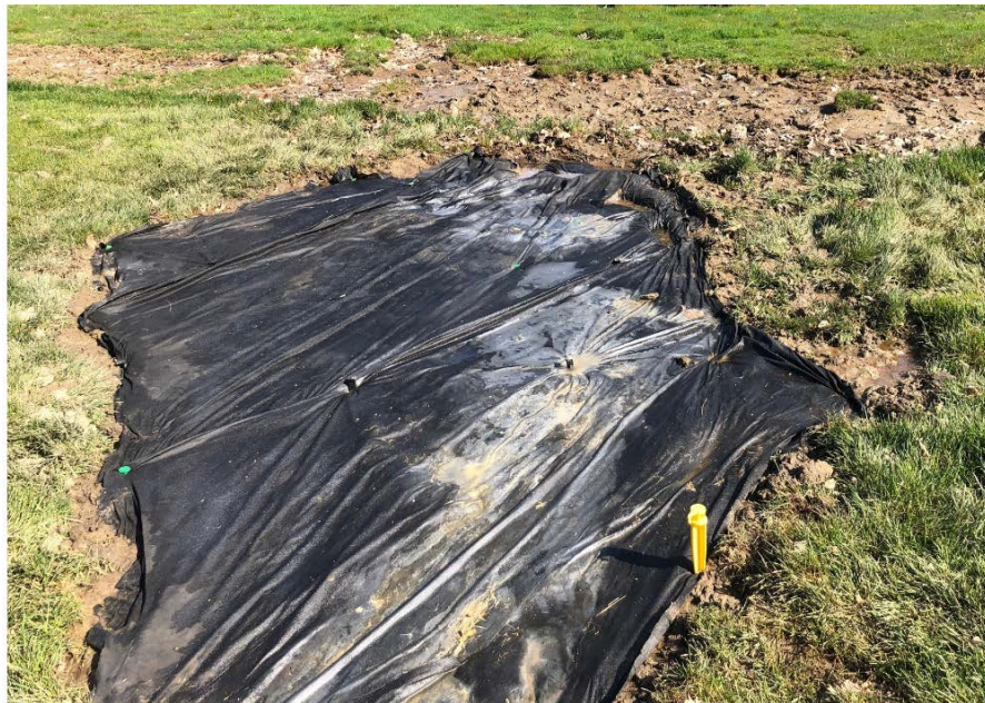
Photograph 2: Precipitate accumulating on filter fabric May 20, 2020
