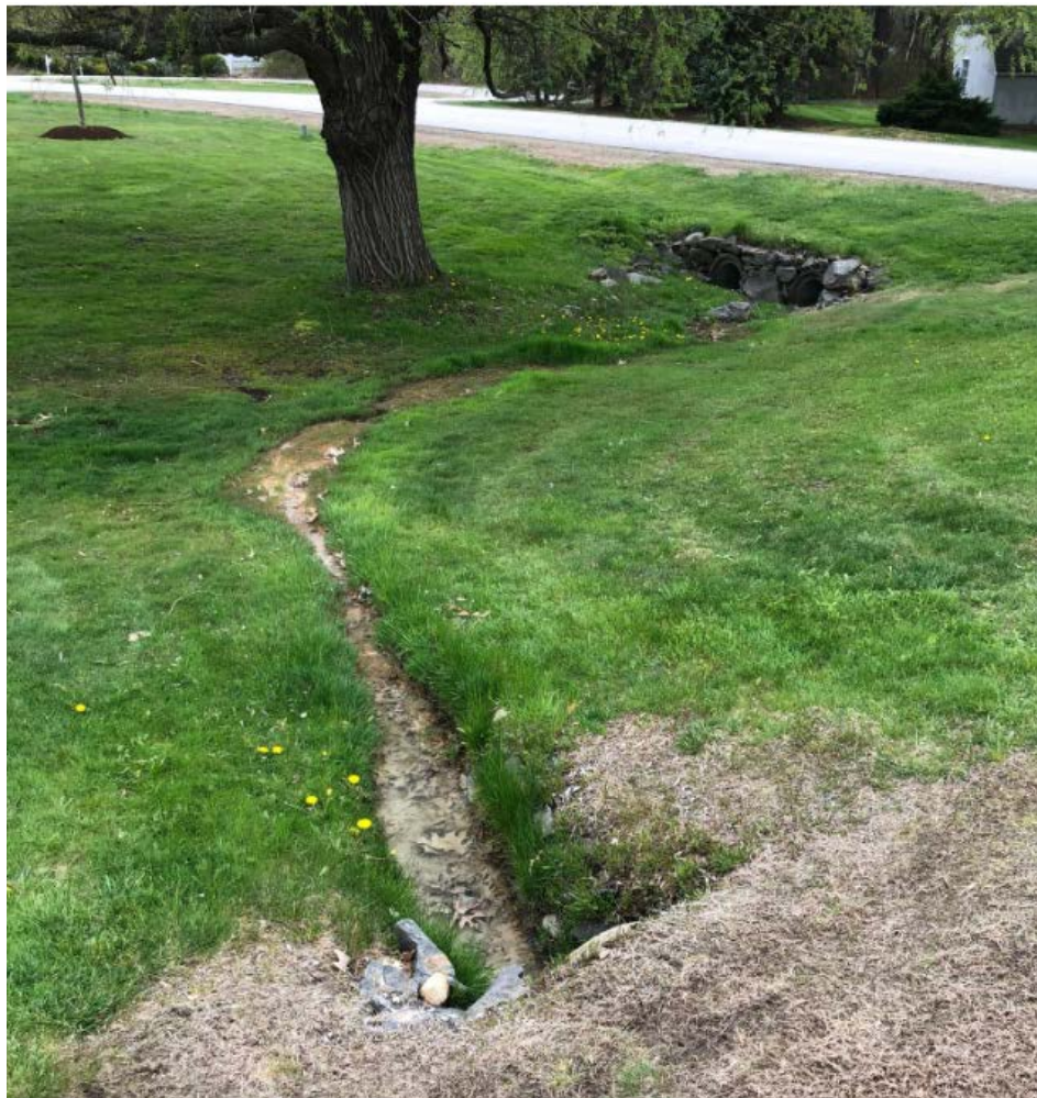
Photograph 3: Drainage Course at Gundalow Landing Culvert Outlet (View facing southwest)
