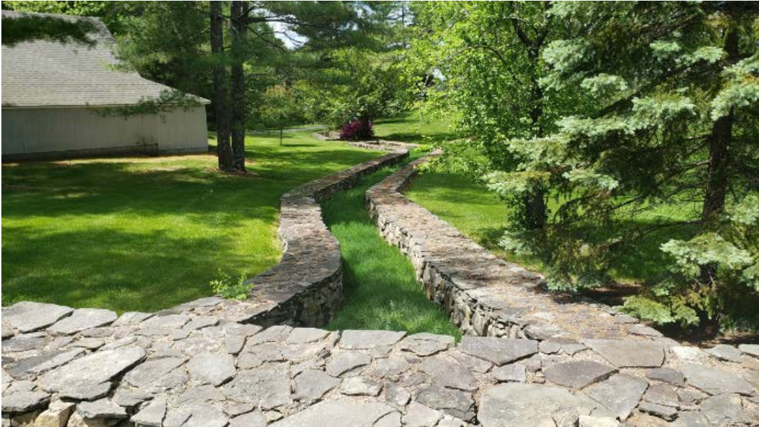
Photograph 4: Drainage course south of Brickyard Circle (facing south)
