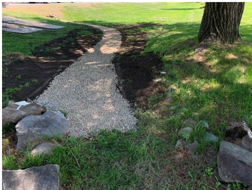
Photograph 6: Drainage course improvement at Gundalow Landing Culvert Outlet (View facing northeast)
