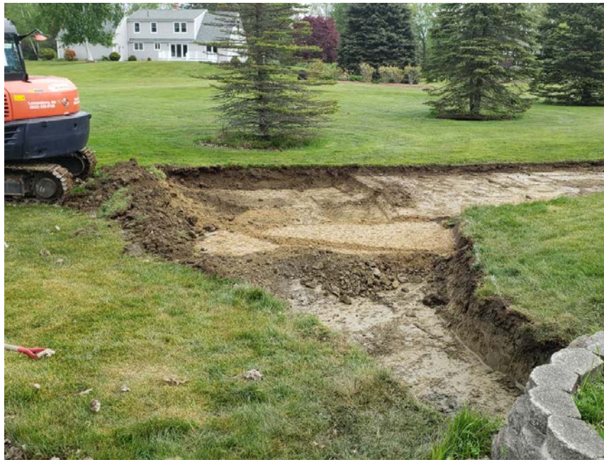
Photograph 5: Excavation of 29 Gundalow Landing Seepage Area in progress
