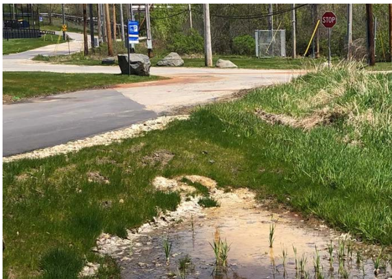
Photograph 9: Precipitate observed south of the Greggs Hall access road
